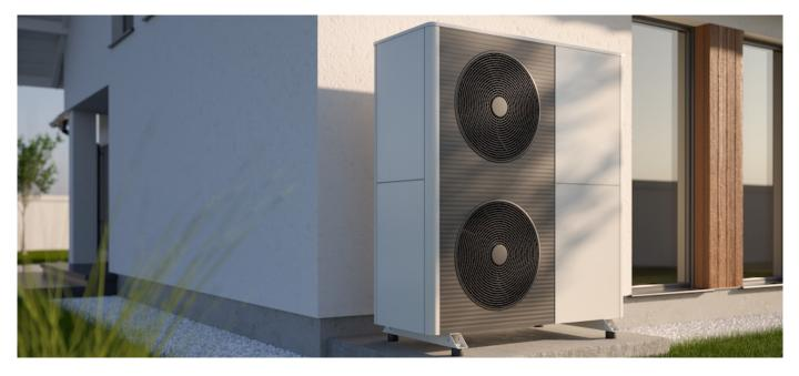
An air source heat pump is slightly larger than an air-conditioning refrigeration unit. They are located outside the buildings and connected to an inside unit through the wall.
